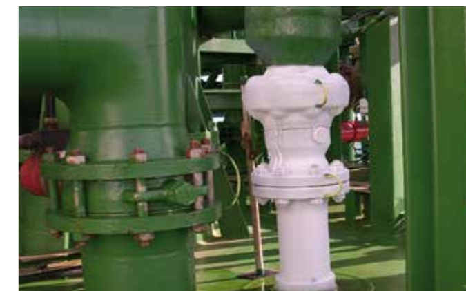
Transporte de amoníaco a baja temperatura Transport of ammonia at low temperature
